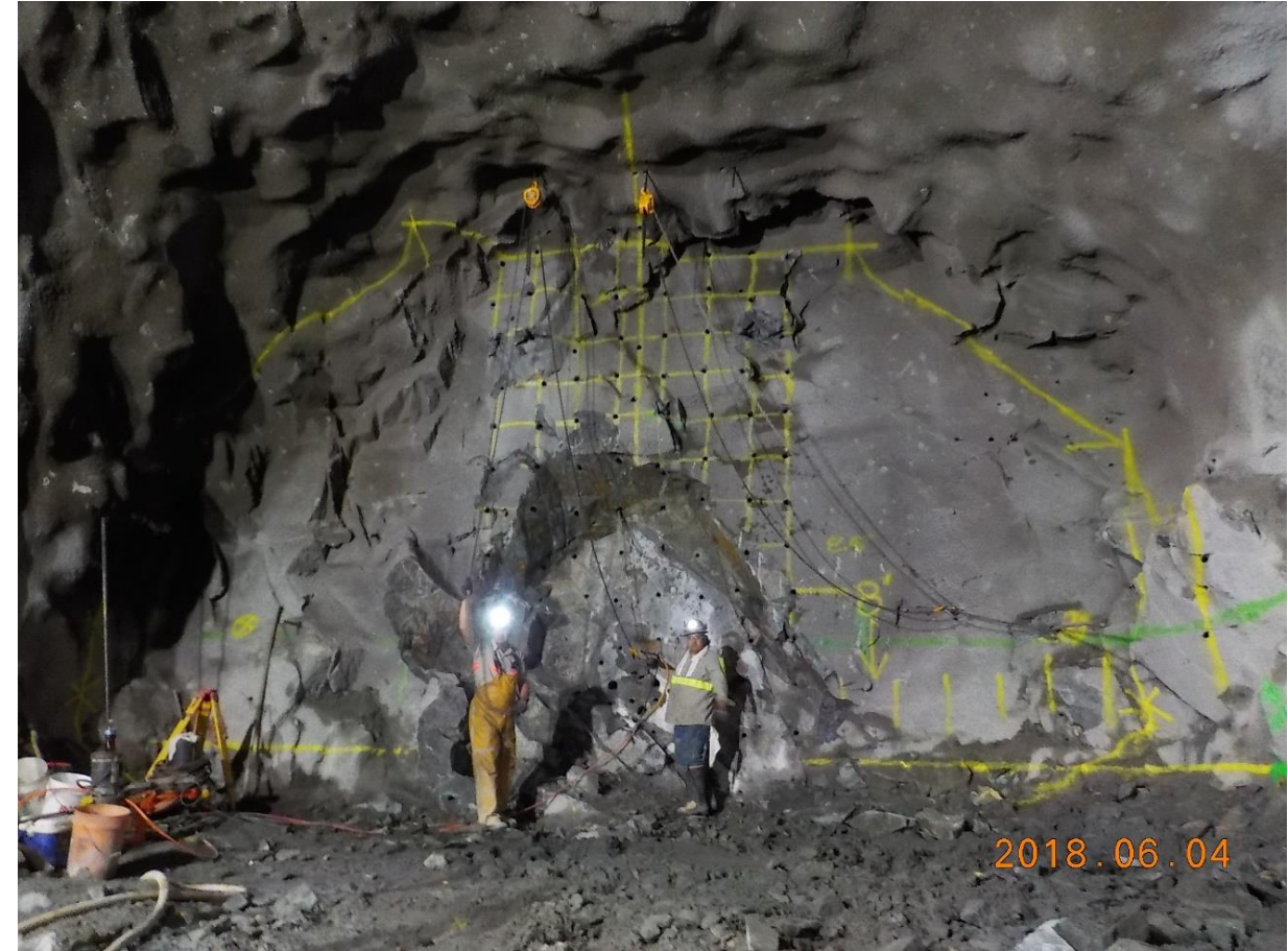
First round of center cut using mechanical excavation
