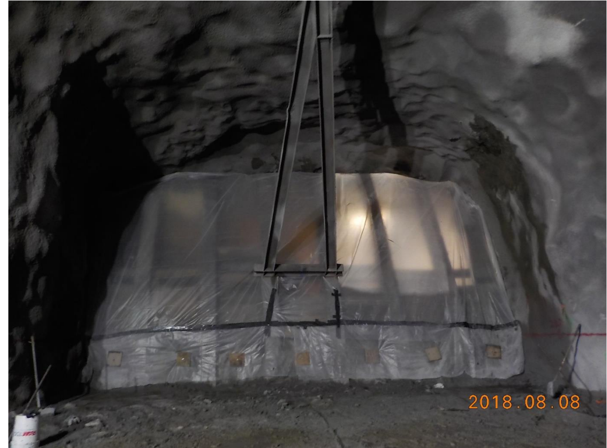
Breakthrough conservation until final support installation
