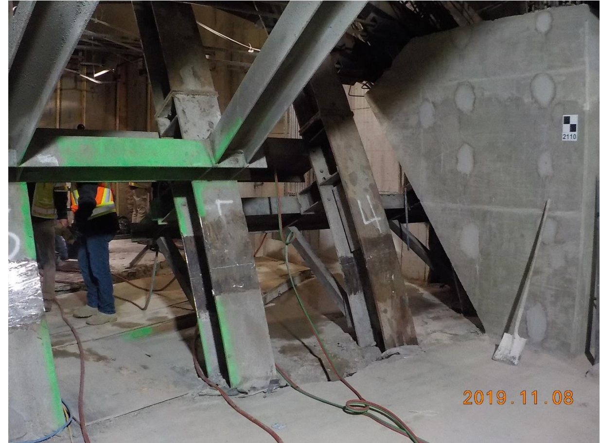
View from tunnel at breakthrough into WMATA station – steel ribs ready for cutting
