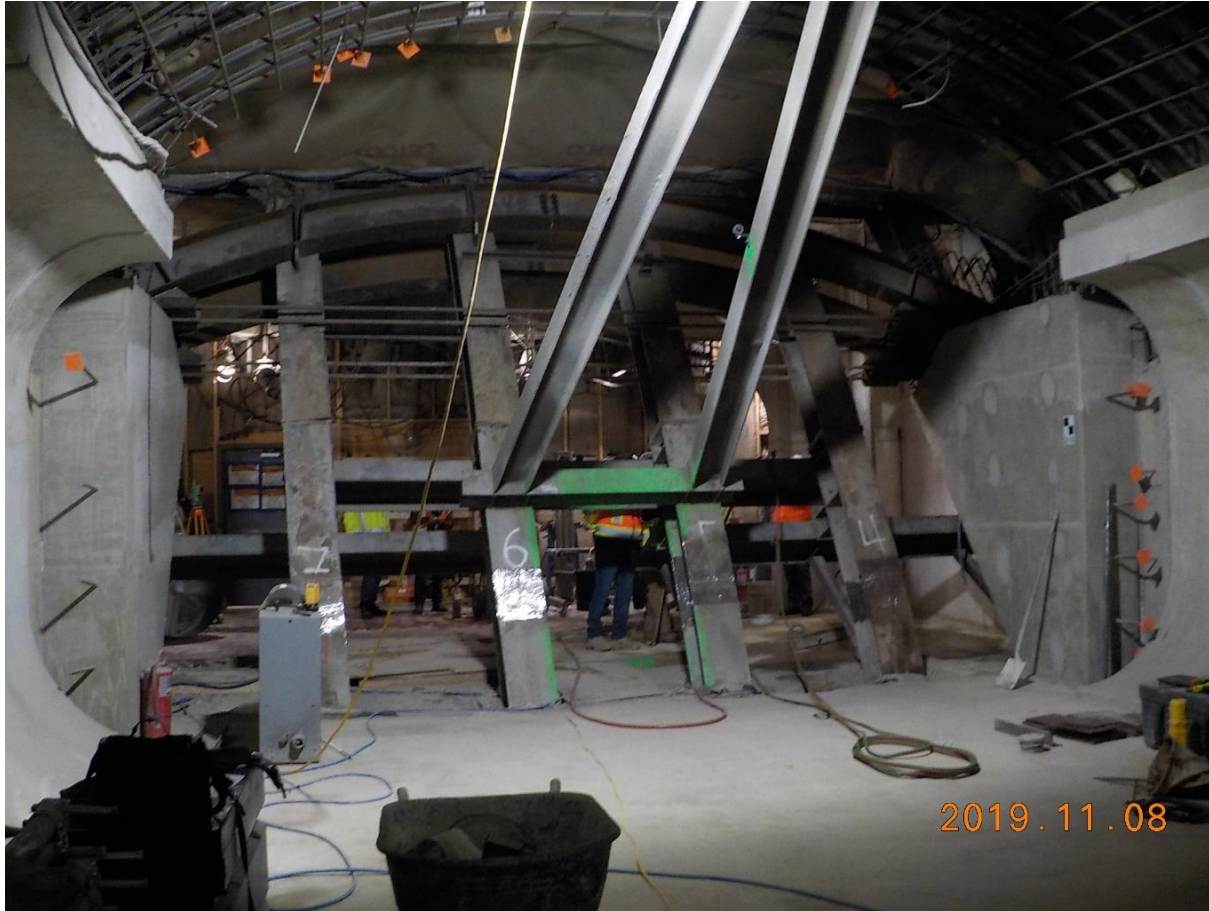
View from tunnel at breakthrough into WMATA station – steel ribs ready for cutting
