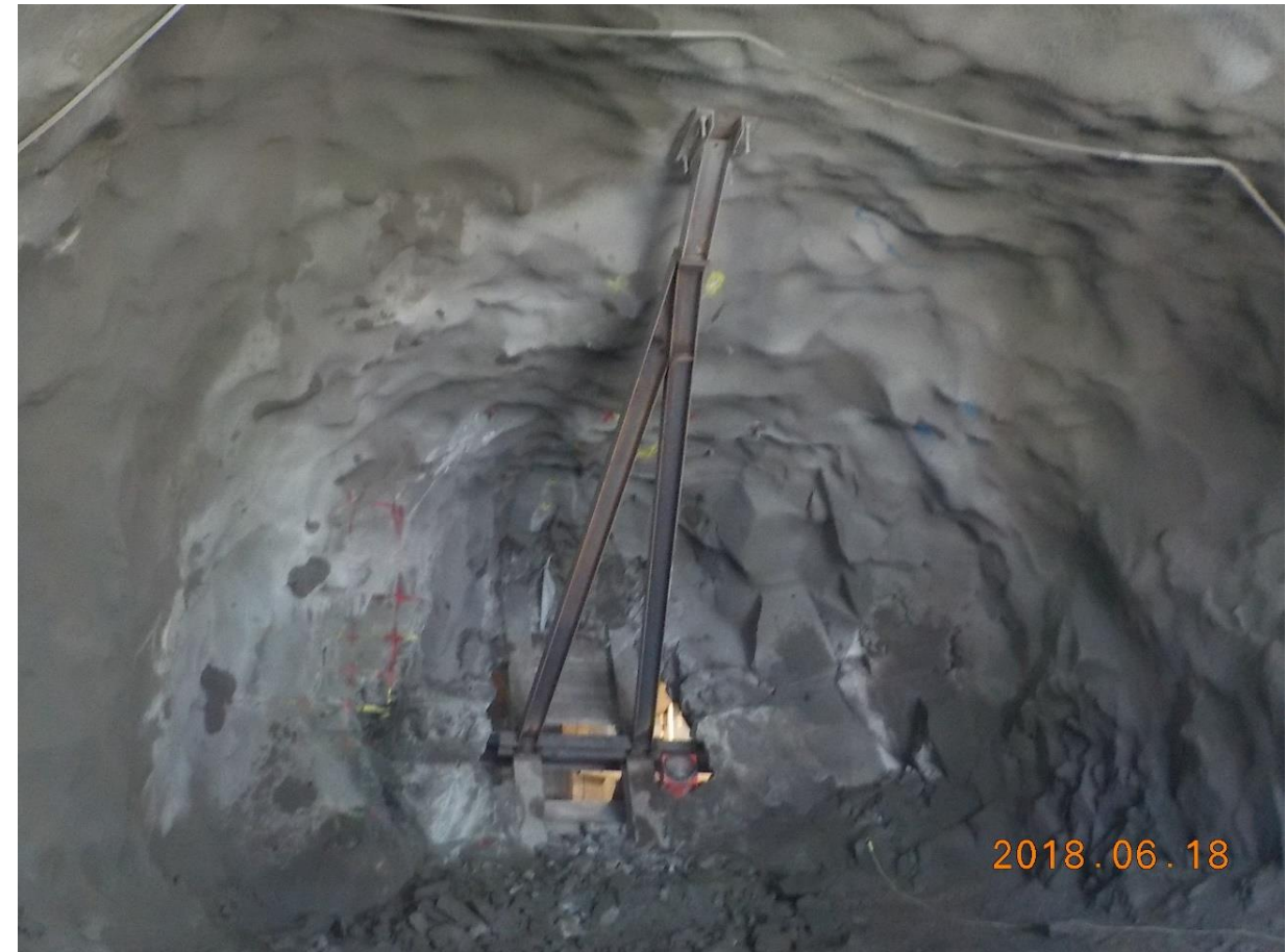
Initial support for breakthrough window
