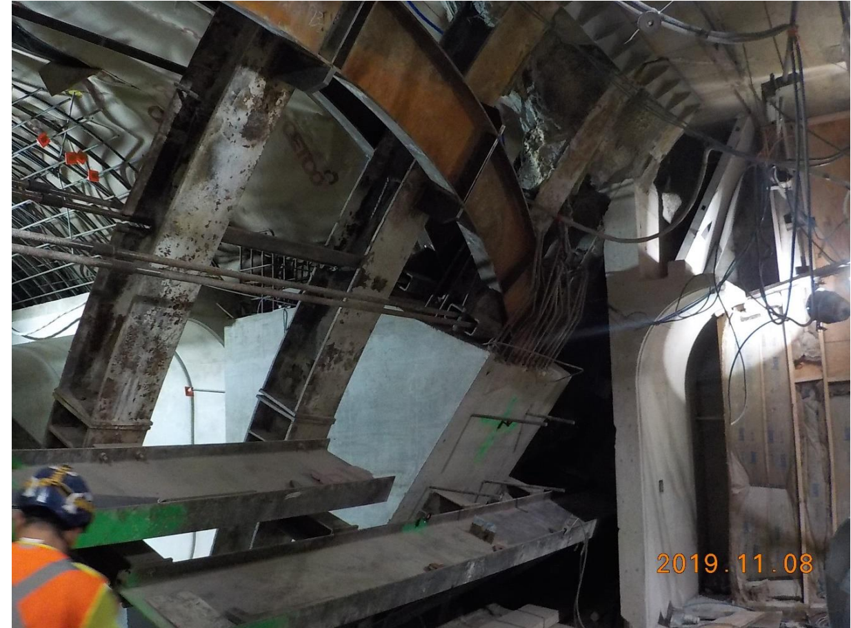
Pickup girder at breakthrough – view from WMATA station into tunnel
