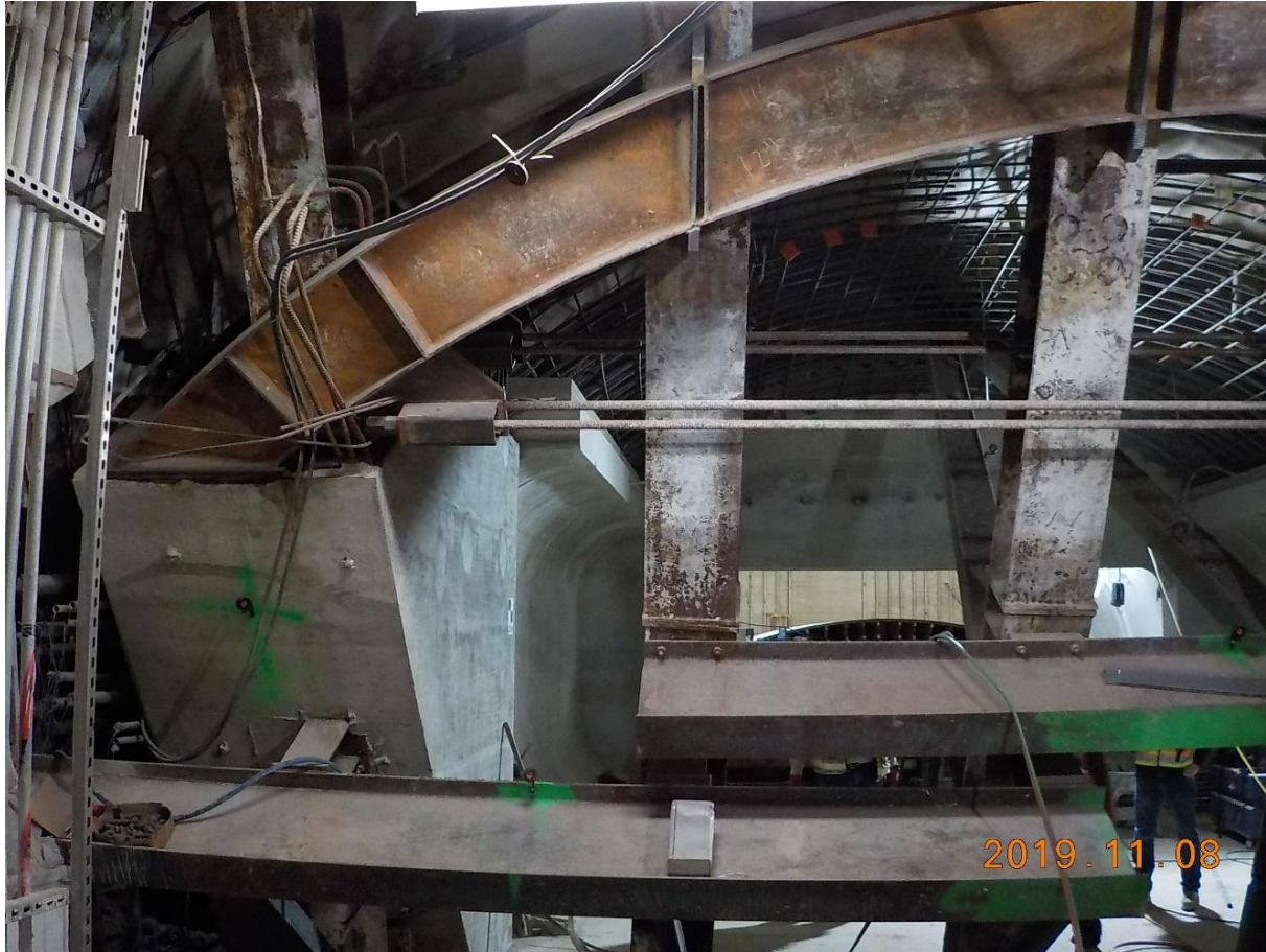
Pickup girder at breakthrough – view from WMATA station into tunnel
