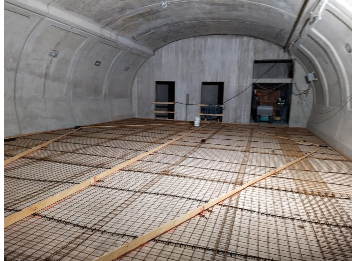
View of the tunnel/passageway after final lining concrete – preparation of topping slab
