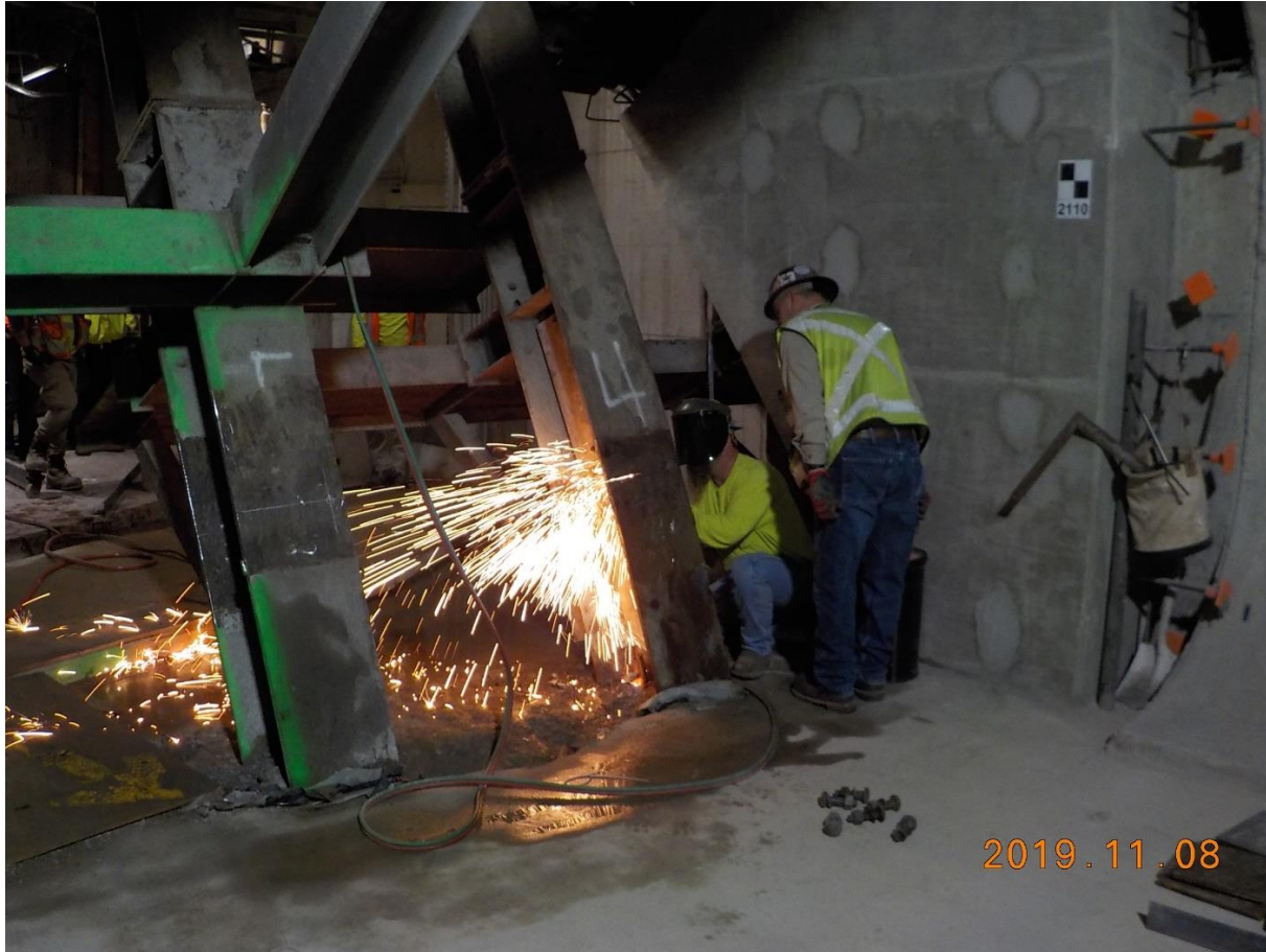
Cutting the lower part of the steel ribs
