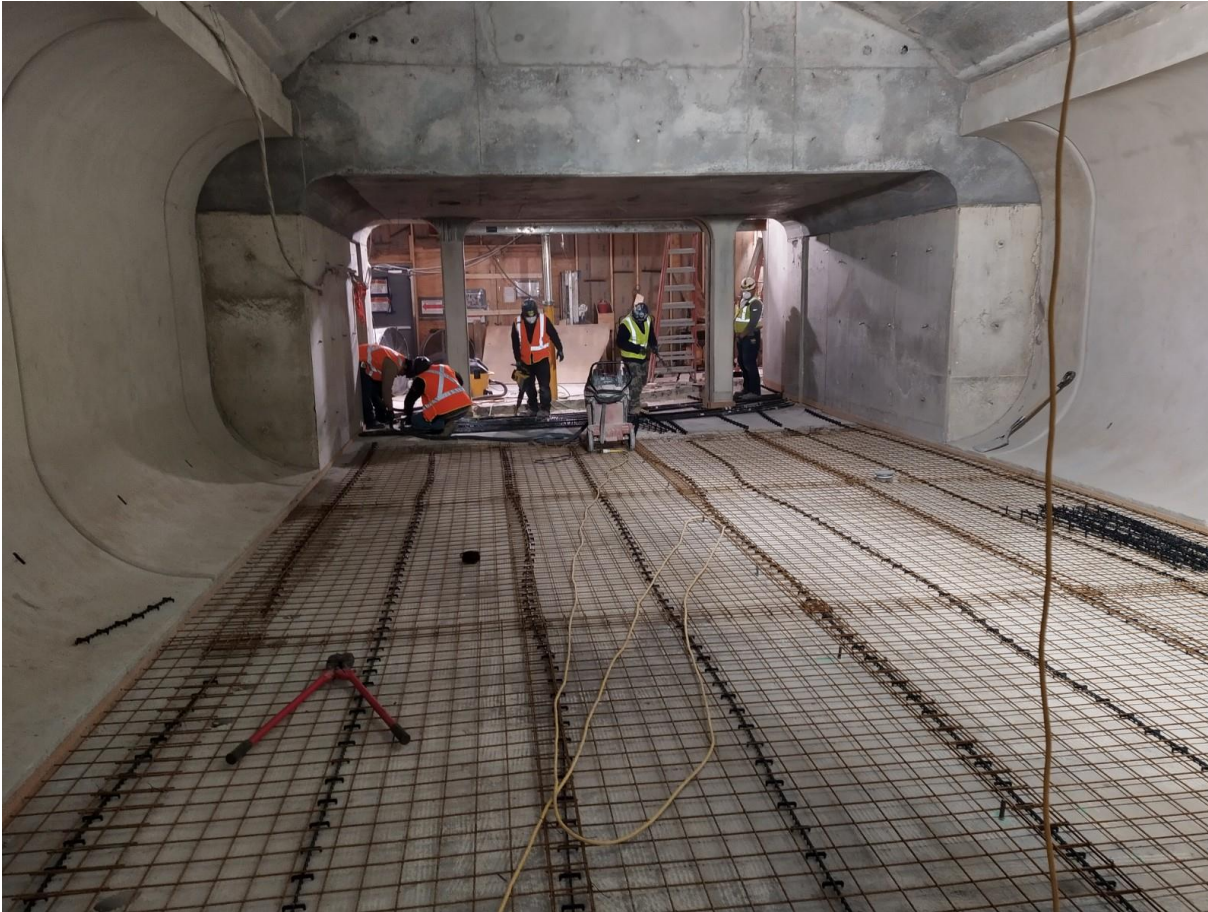
View of the tunnel/passageway after final lining concrete – preparation of topping slab
