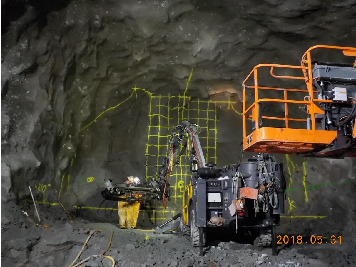
Drilling center cut for mechanical excavation
