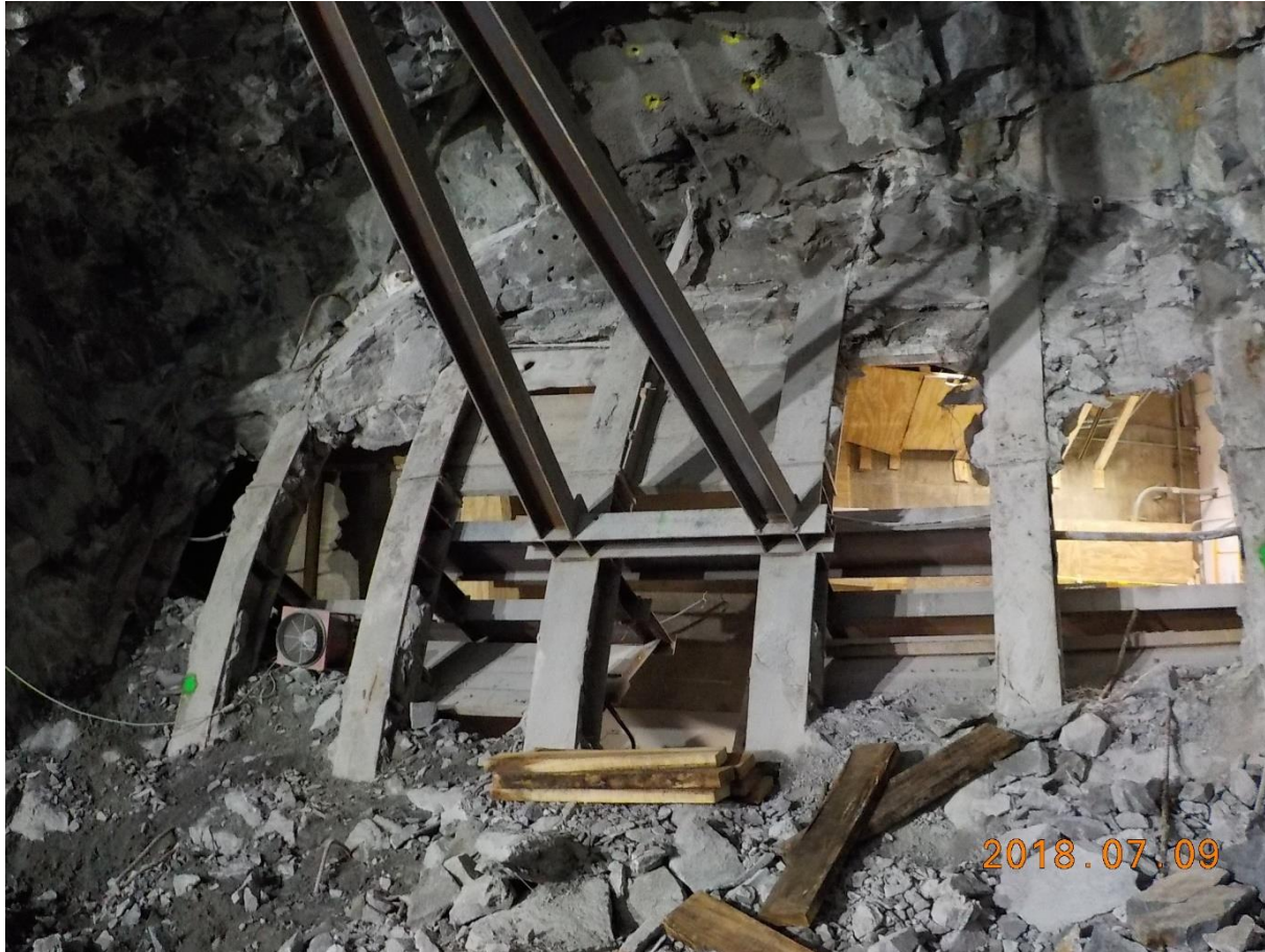
Full set of steel ribs exposed
