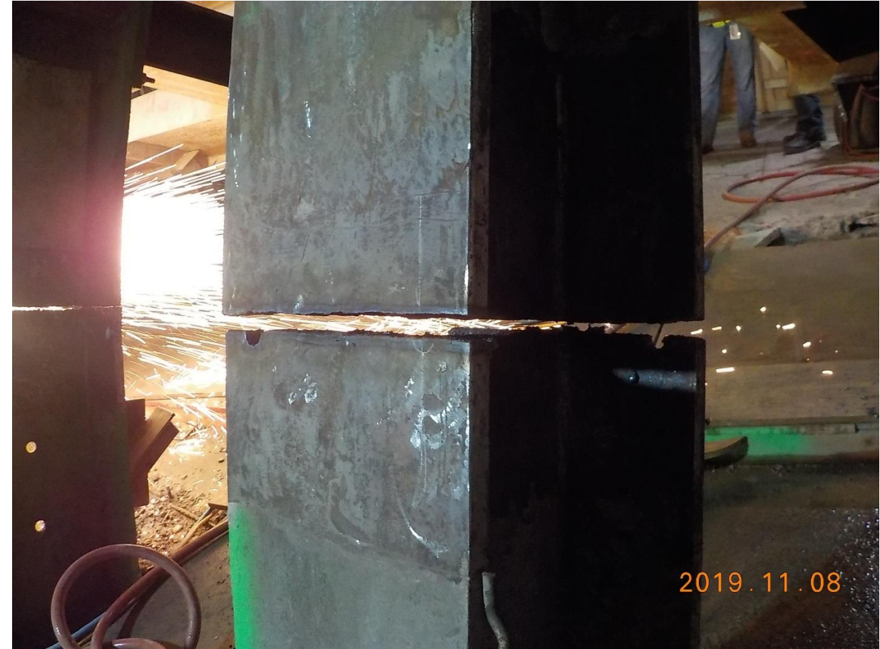
Cutting the lower part of the steel ribs
