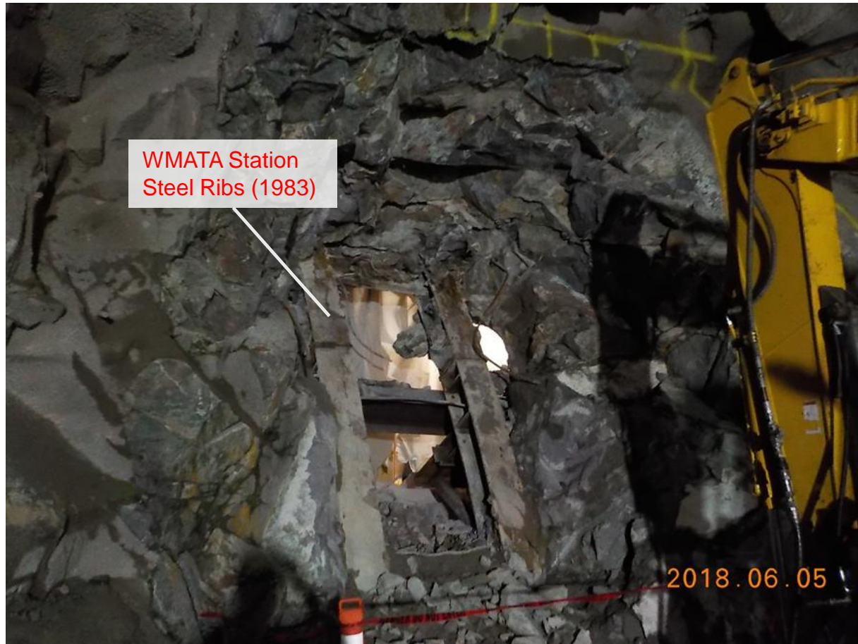
Breakthrough window into WMATA station
